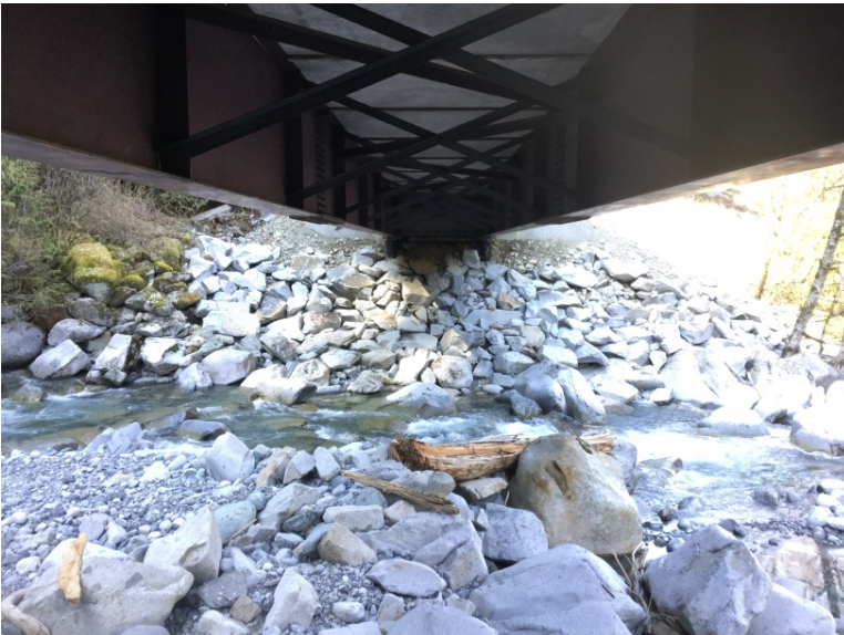
Left Bank Abutment when facing downstream
