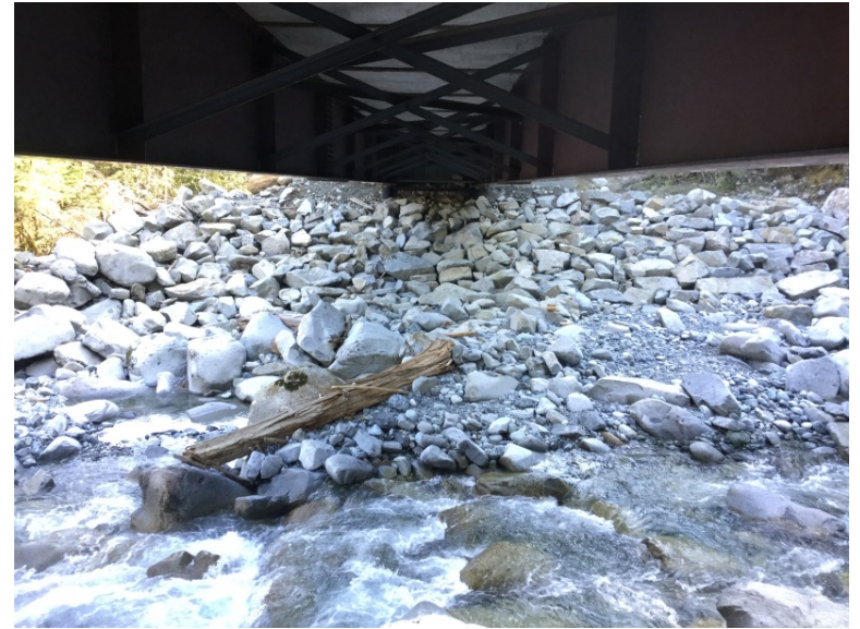
Right Bank Abutment when facing downstream
